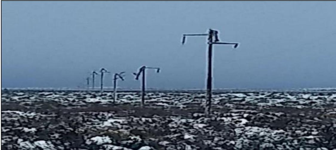
*Fig. 34 - Torres colapsadas LAT-132 KV tramo Cutral Co-Zapala*
