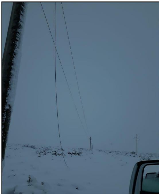
Fig. 36 - Torres colapsadas LAT-132 KV tramo Cutral Co-Zapala
